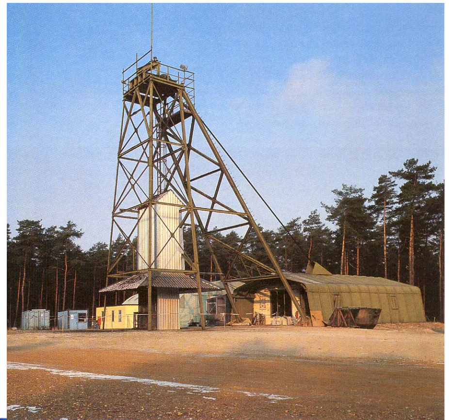
View of the first shaft
